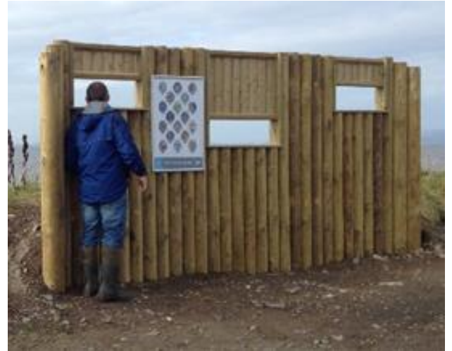
(Above) Viewing screen example - this one is robust for use in an exposed environment - screens the viewer from species which may flee from disturbance, slots at different heights for people of varying heights and abilities – identification chart to help
